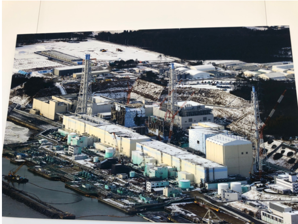
Undated photo of 4 reactors, here with Reactor 1 (at right) covered. The cover was installed in October 2011 but the roof was removed in 2015, while the wall panels were removed in 2021 in preparation for installing a new building cover in 2023 to facilitate spent fuel rod removal. The other three reactors are now all shrouded (see below). Credit: The Great East Japan Earthquake and Nuclear Disaster Museum.
