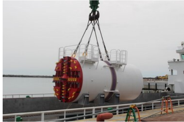
Water discharge system under construction. April 2022. Credit:TEPCO
