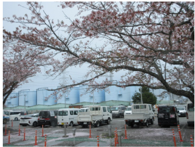
Water storage tanks at Fukushima Daiichi, April 2022. Credit: TEPCO
