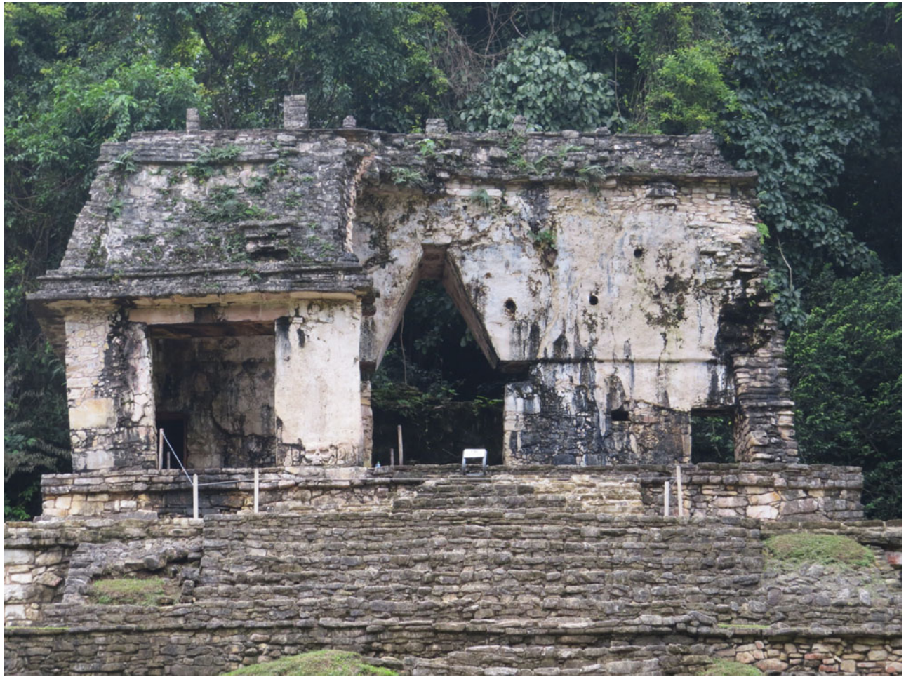
Figure 5. The cross-vault encompasses the central door in Temple XII's central wall. Photograph courtesy of Esteban Mirón Marván.
