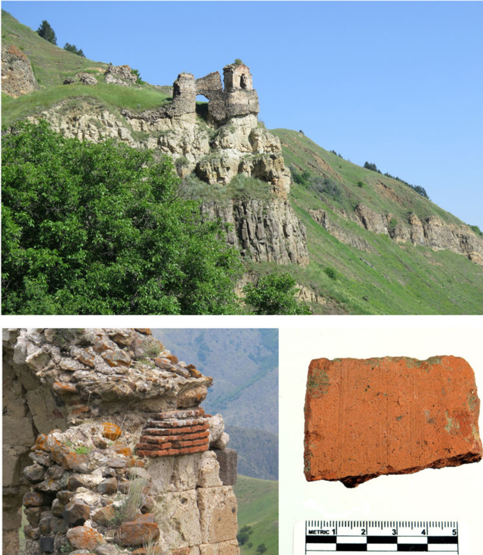
Figure 11. Varneti church (a) view from the south; (b) tiles built into the apse wall; (c) tile from the surface at Varneti hillfort.
