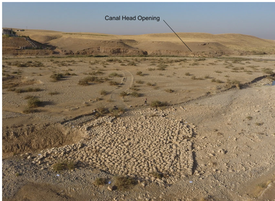
Fig. 21 The Neo-Assyrian dam across the Bastora River, with the subterranean channel entrance in the background. UAV photograph taken 30 September 2016.
