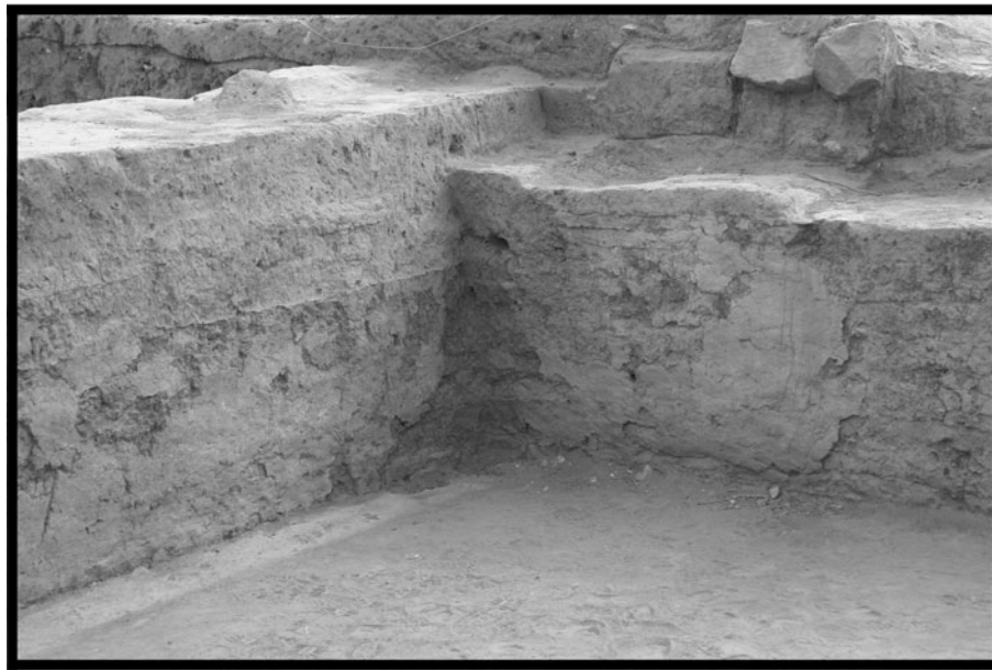
Figure 5. Example of adobe walls in Edificio 4 with mud and lime coating. Note the stucco floor. Photograph by Dan M. Healan.
