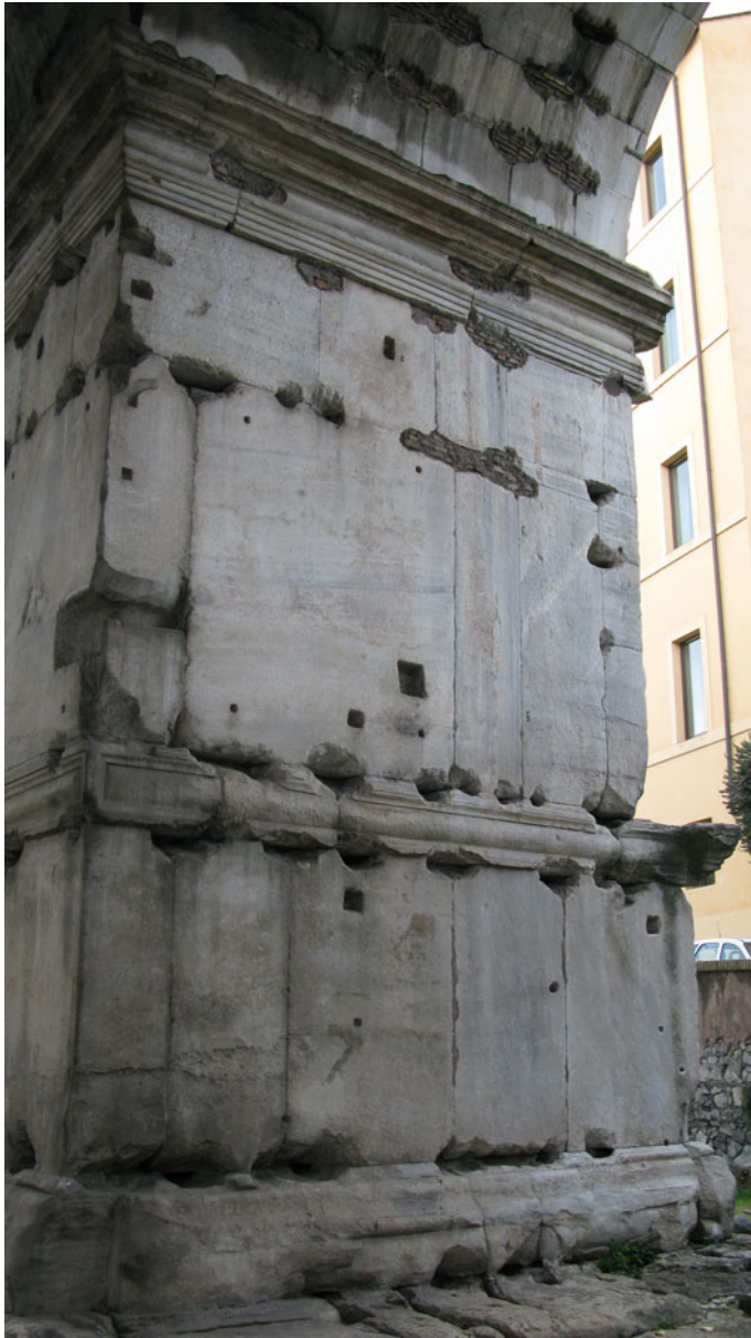
FIG. 7. Detail of the new cornices created for the Arch of Janus.
