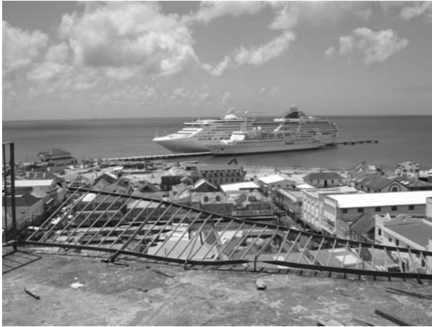
View from roof of Sir Archibald Law Library, St. Georges, Grenada showing houses with plastic sheeting, but cruise liners Oceania and Delphin returning.
