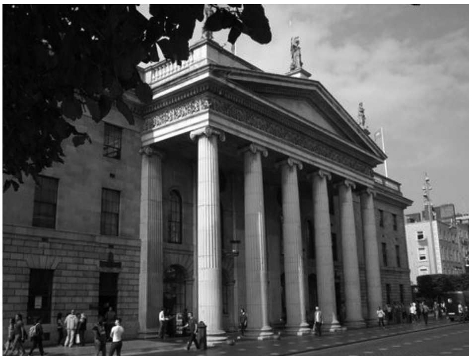
Figure 4: General Post Office, Dublin. The revolutionaries who founded the Irish Free State following the Anglo Irish Treaty of 1921 had a pragmatic streak. While asserting nationhood and independence, they largely preserved the political, judicial and administrative structures that existed prior to independence.
