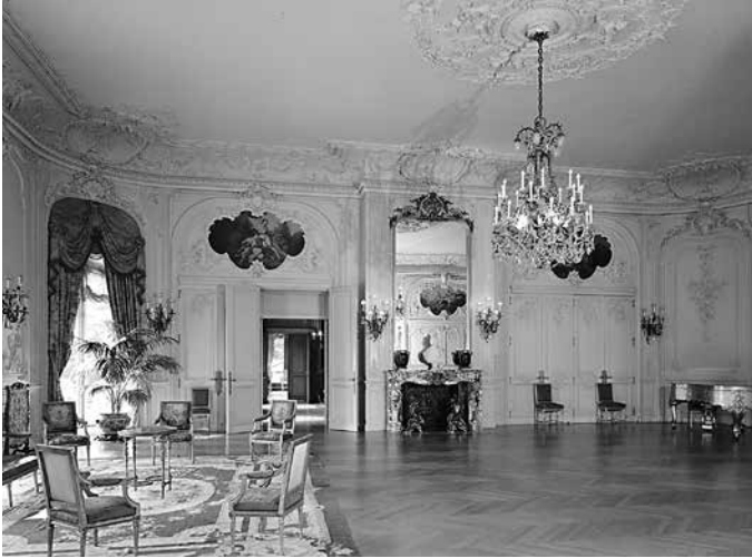
Fig. 6. The Elms , Newport, Rhode Island, Horace Trumbauer and Jules Allard, 1899–1901, Ballroom, photograph by Historic American Buildings Survey, after 1933 (Library of Congress, Washington DC)
