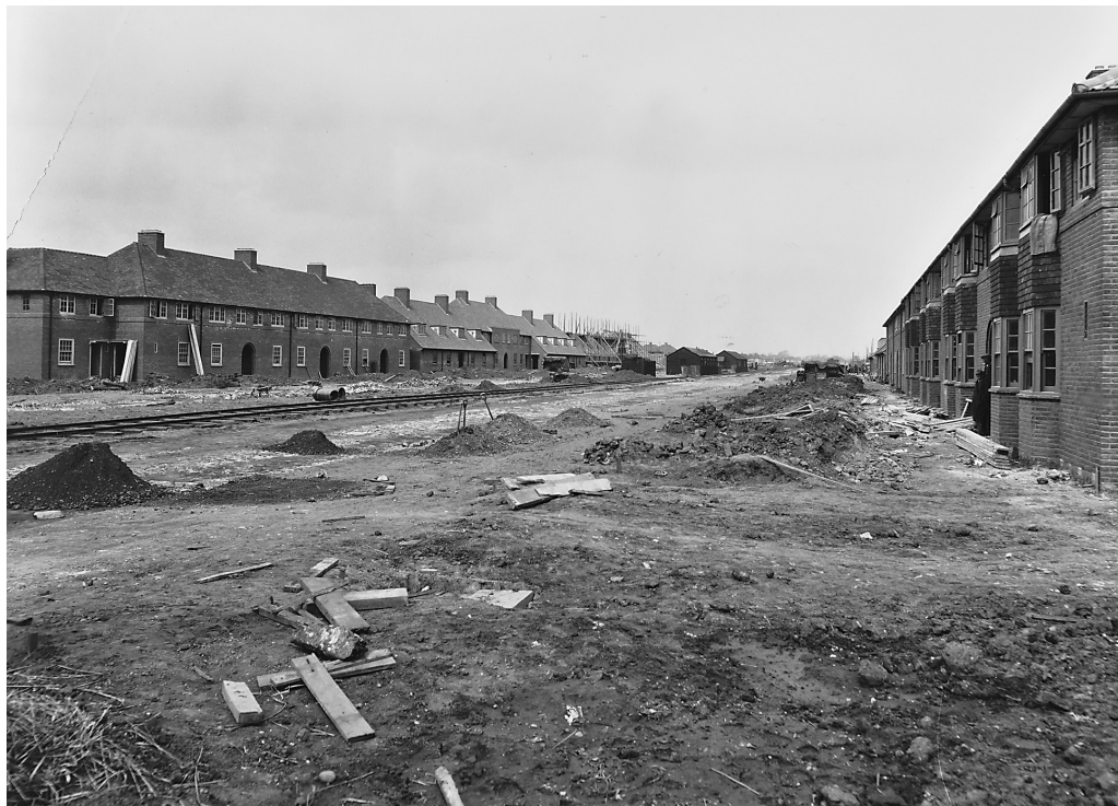
Fig. 8. Construction work in progress at Becontree, photograph of 1925 (London Metropolitan Archives)
