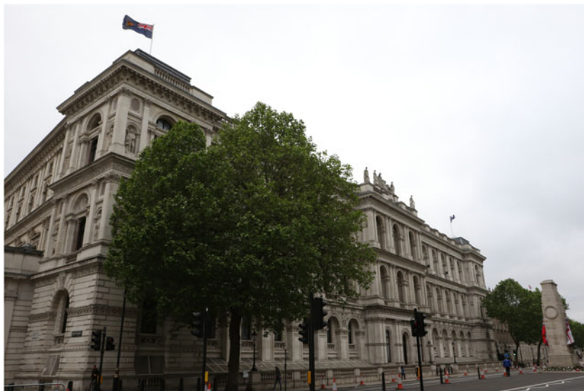
Figure 1. The FCO building from Whitehall.
