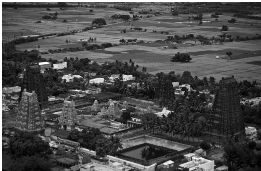
Figure 2. Aerial view of the Bhaktavatsala temple, Tirukkalukundram
