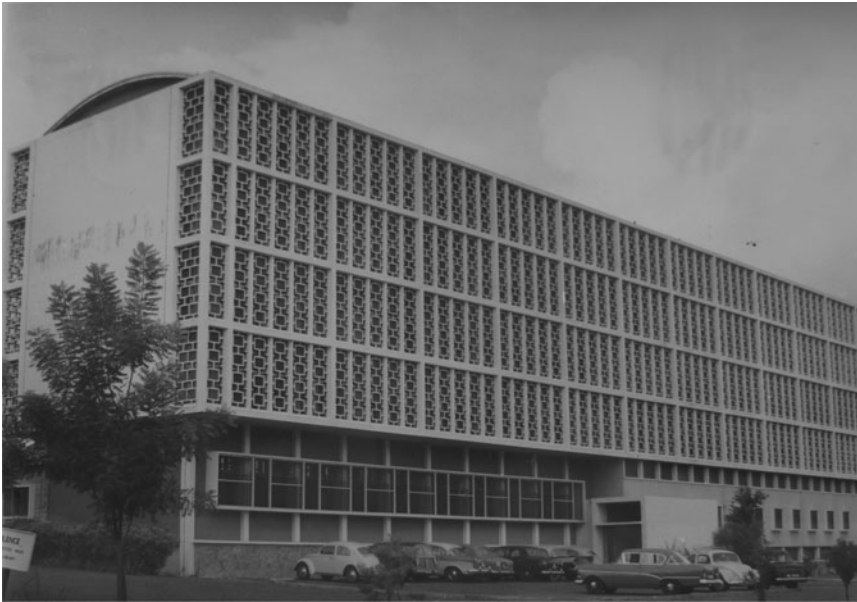
Figure 3: UCI Library. Note the perforated concrete screen, which allowed the natural ventilation of the building, but also let in noise. The sign in the bottom left corner reads, 'SILENCE REQUESTED NEAR LIBRARY'.
