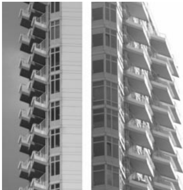
Figure 3 (Zaidi & Griffiths). (Left) A view of the apartment building “The Future,” located at 200 East 32nd Street in New York City. The balconies appear to tilt up, with tilt becoming more apparent the higher up the building one looks. (Right) The same building, but viewed from the opposite side. The balconies now appear to tilt downwards.
