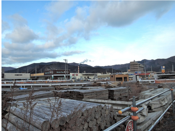
Reconstruction near the port of Ōfunato. Photo by the author, February 2016.
