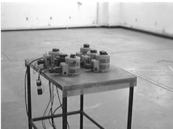
Figure 4. Six control rheostats on table with replaced floor in the background.
