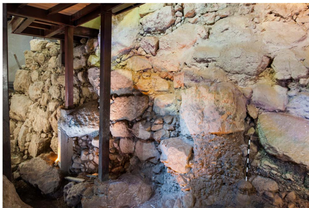
Figure 3 Photograph of the outer face of the Spring Tower (Wall 104), with unfinished boulders and plaster partially coating the stones.
