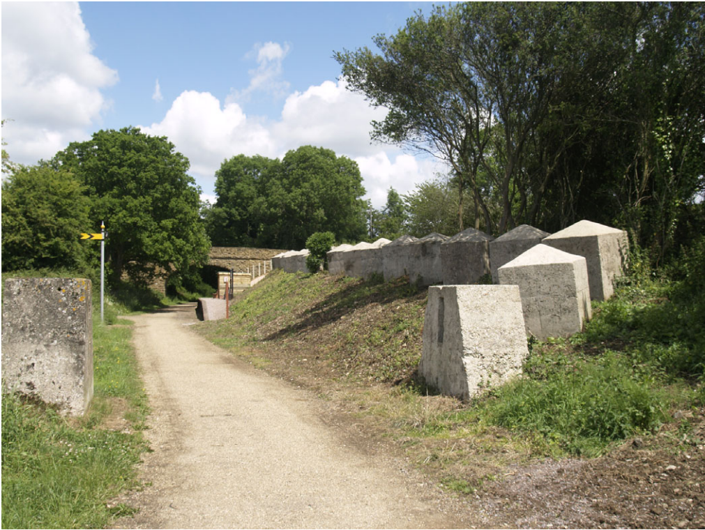
Fig 2. Taunton Stop Line defences at Donyatt in 2009 looking north. The stop line followed the railway, then in use, with an anti-tank ditch on the west side (HER 11063). The obstacle crossed the line at the railway block (HER 55412) in the foreground and was then carried up to the bridge by concrete cubes (HER 55355) to another roadblock (HER 55356) across the lane before continuing north on the east side of the railway cutting. The former railway halt has been reconstructed as an information point on a cycleway and the concrete cubes (and one side of the railway block) cleaned. This provides an impression of the situation when the concrete was newly cast and shows the need for camouflage, if only in this case by paint or dirtying. Photograph: Somerset Historic Environment Record.
