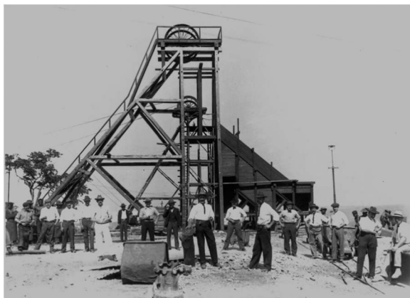
Figure 4. Ayrshire mine, main shaft headgear. It was 68 feet high, built of imported pitch pine, and equipped with three-ton and one-ton skips. Source: National Archives of Zimbabwe.
