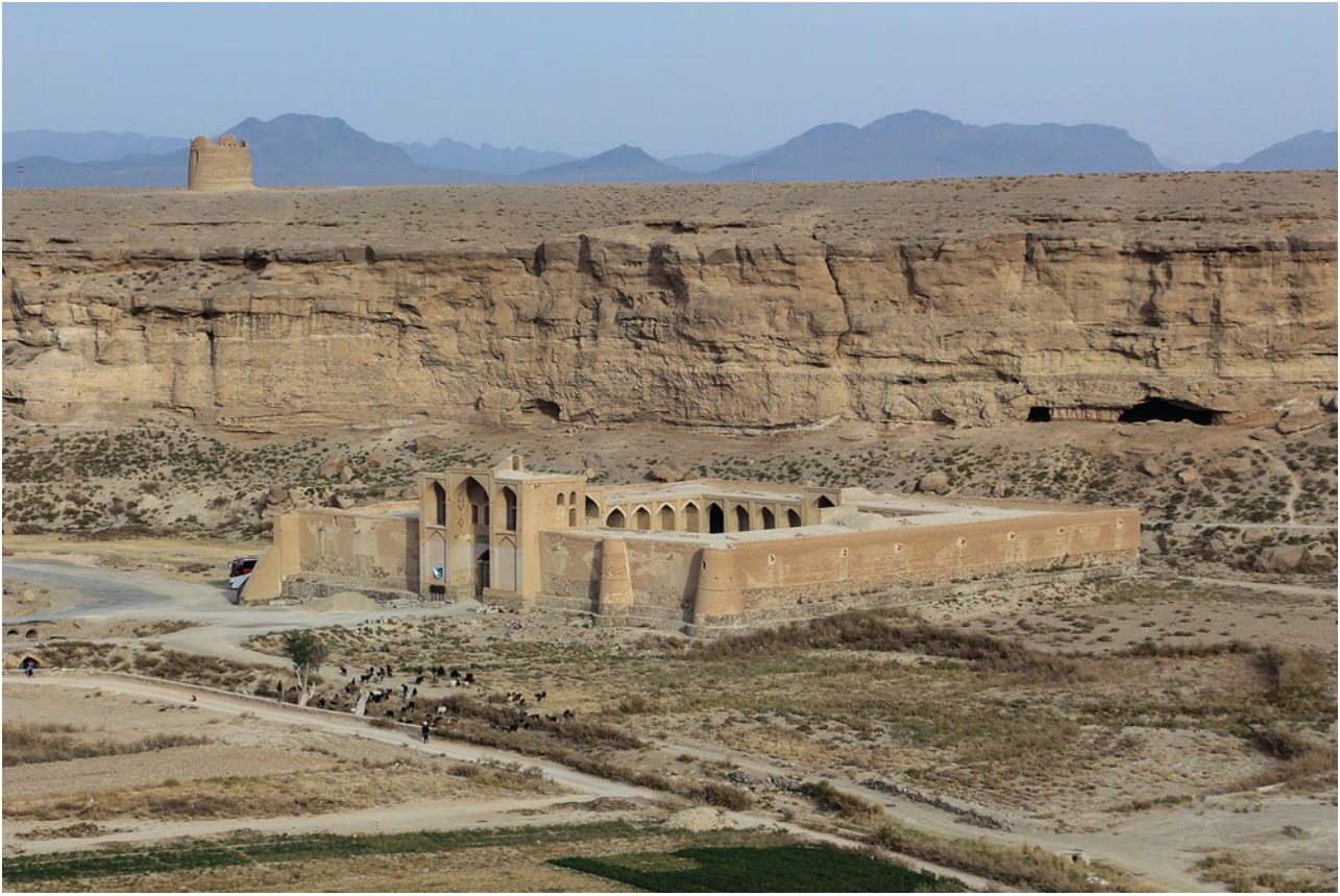
Figure 2. Example of rural caravanserai stopover, landscape shrines, and fortified public area, Fars Province, Iran: Izadkhast caravanserai, seventeenthth century. (Photograph: Bernard Gagnon, Wikipedia commons.)
