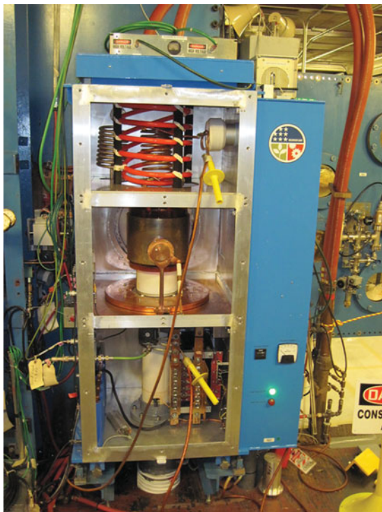
Fig. 4. New FPA cabinet. It has the same dimensions and is designed to operate with the existing signals and resonator structure, allowing testing it in a reversible way. The filament power supply is integrated in the new cabinet for convenience.
