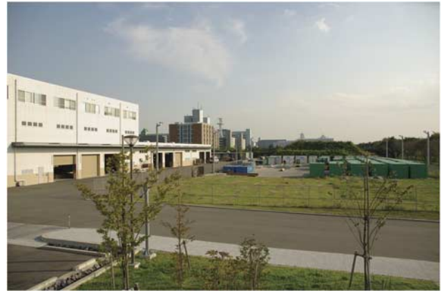
Fig. 1. The location of the warehouse, the cargo handling area and the container yard of the National Institute of Polar Research (NIPR) in Tachikawa-shi.
